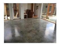
Burnishing is used for maintenance, rejuvenating and removing mechanical or chemical damage.
